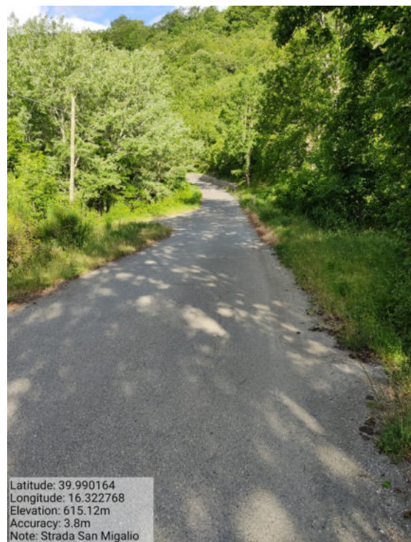
Int. _6.3_ Manuten. Strade Loc. San Migalio Foto 2
