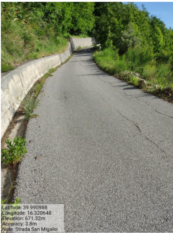
Int. _6.3_ Manuten. Strade Loc. San Migalio Foto 1
