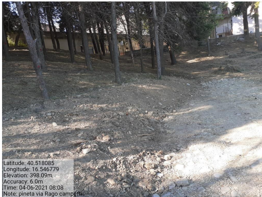
Intervento 2.1.1 Area Urbana Pineta Via Rago — POST OPERAM
