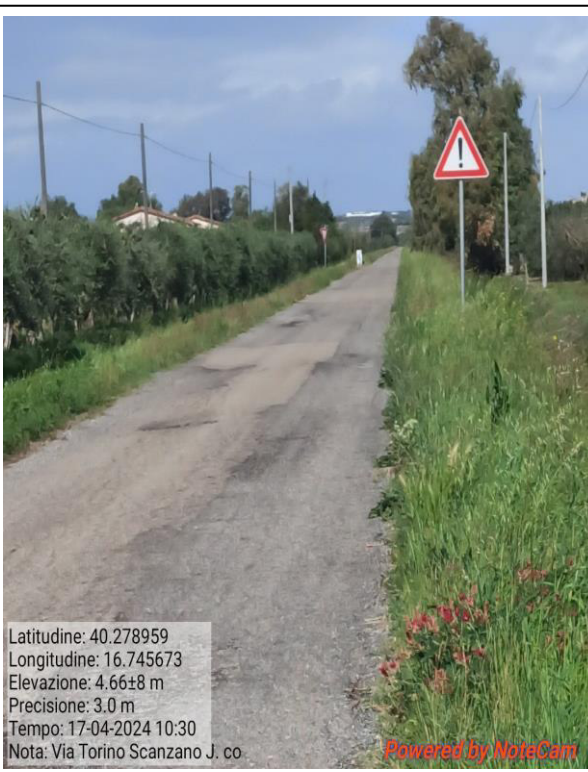
Int. 6.3.11.1 Via Torino Decesp. scarpate stradali
